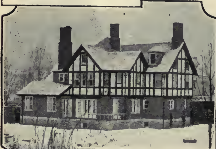
Residence of J. M. G. Brown, Morgantown, W. Va. Adscos Heating.
